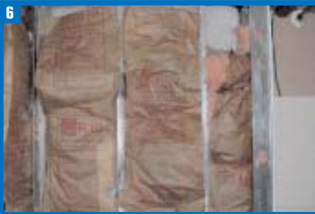
(6) Typical light-weight metal wall studs and insulation used in today's construction.
