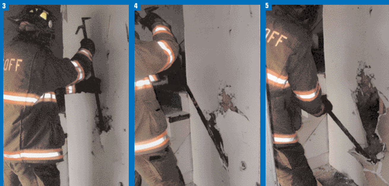
(3) The firefighter slides the hook's handle down into an entry hole. (4) As he pulls the hook's handle toward the floor, he opens up the wall. (5) Be prepared for the drywall to break up into small or large pieces when using this technique to open up walls.
